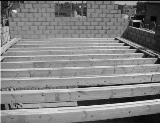
A black and white photograph showing the wooden beam floor construction of a building. The floor consists of several parallel wooden beams supported by a brick wall on the right and another wall on the left. The beams are laid out in a grid pattern, ready for a floor finish. |
