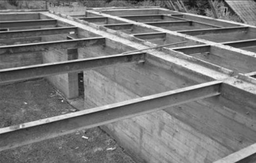
A black and white photograph showing the metal beam floor construction of a building. The floor consists of several parallel metal beams supported by a brick wall on the right and another wall on the left. The beams are laid out in a grid pattern, ready for a floor finish. |
