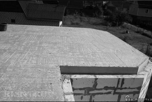
A black and white photograph showing a monolithic concrete floor. The floor is a single, continuous slab supported by a brick wall on the right and another wall on the left. The floor has a textured surface.                                                                    |
